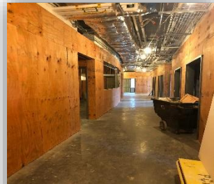
Preparations for drywall work continues with the installation of plywood in the ED.
